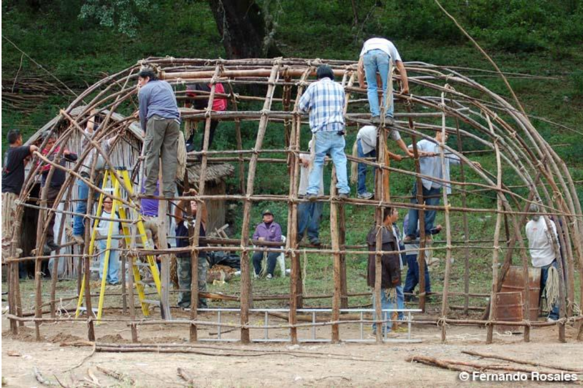
Construction of a traditional Kickapoo winter home, 2005. Coahuila, Mexico. Photo by Fernando Rosales; courtesy of the photographer.
