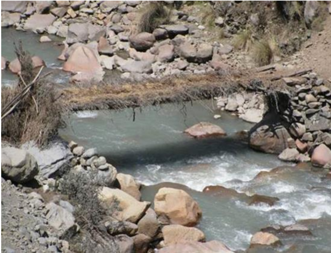
Caption: Plank bridge in Quella Quella, Peru. Photo by Ramiro Matos, NMAI, 2009.
