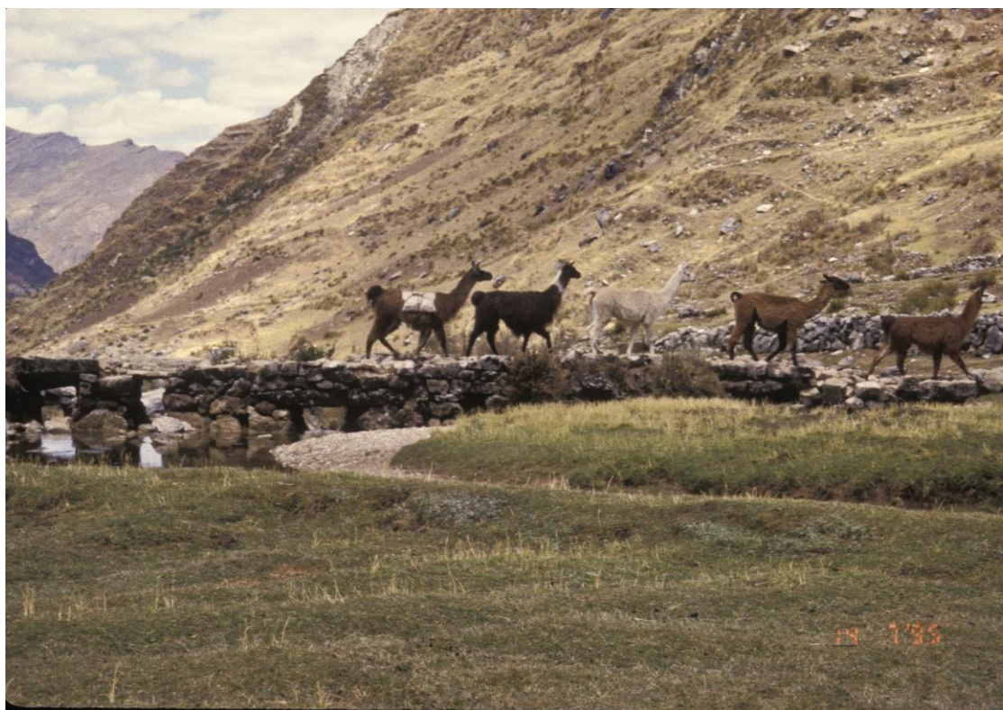
Caption: Inka culvert bridge over the Warautambo River near Warautambo, Peru. Photo by Ramiro Matos, NMAI, 1984.
