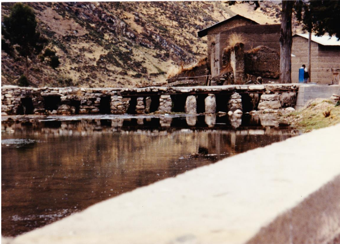
Caption: Inka culvert bridge in Lauricocha, Peru. Photo by Ramiro Matos, NMAI, 1984.
